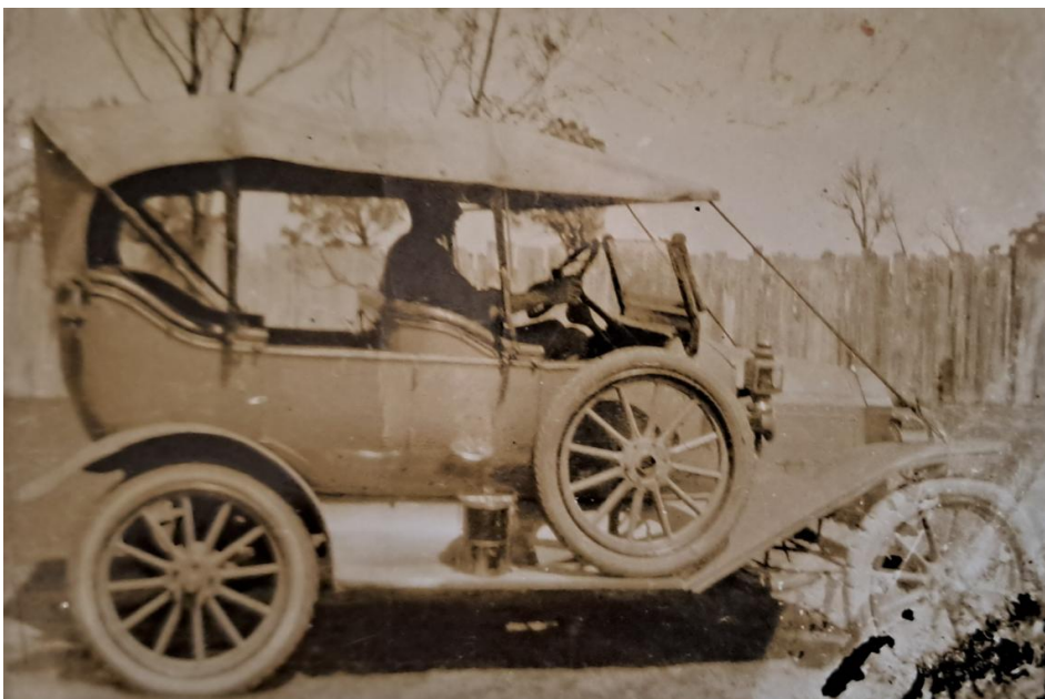
Another side shot of the Ford showing the acetylene generator on the running board that provided flammable gas to the head lights.
